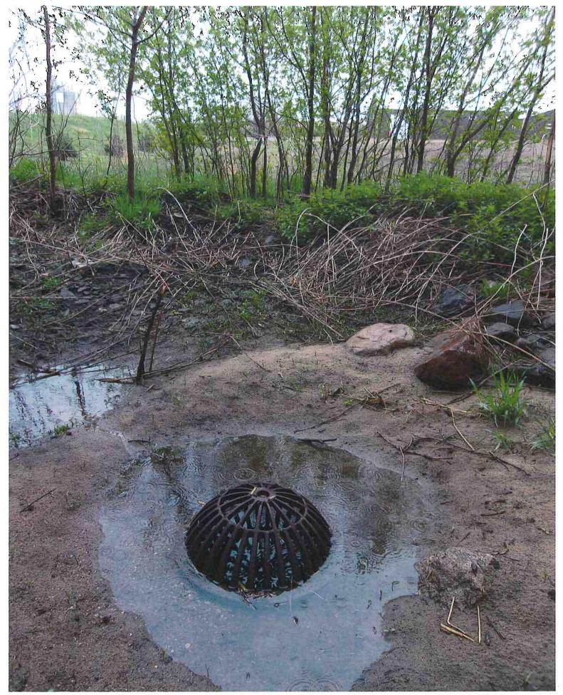
THE HAS BEEN PARTIALLY RUGGED FOR SOMME TIME LOOKING DOWN STREAM, NOTE ALL SEDIMENT SAND BLOWN OUT OF INTAKE
